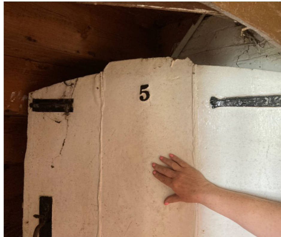
Above left - 17th century cellar door with blacksmith made hinges and shaped top. Above right – mortice holes in the underside of the purlin made from re-used timber close to the eastern dormer and round wood timber used to infill timber frame.
