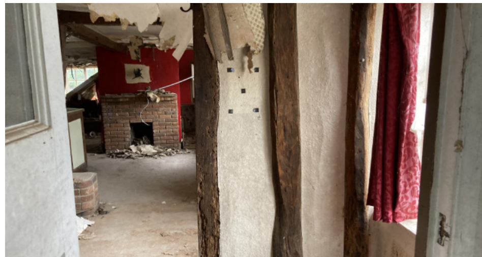
Historic pieces of timber help form a draft screen but do not join into the timber frame and cut across one window.
