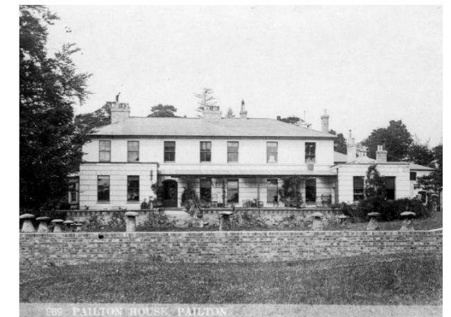
Pailton House and Gardens. 1910s
