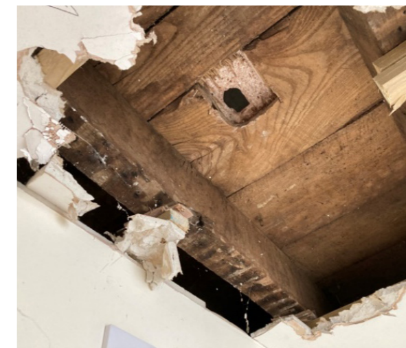
Limecrete over elm floorboards to create some sound proofing between the attic rooms and the bedrooms below.
