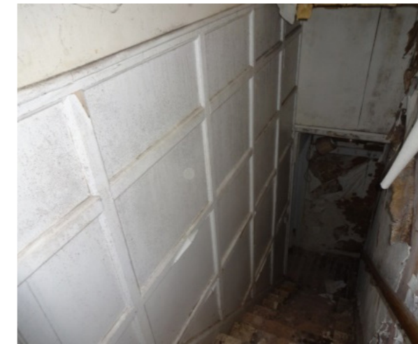
Panelled stair access to upper function room c. 1850
