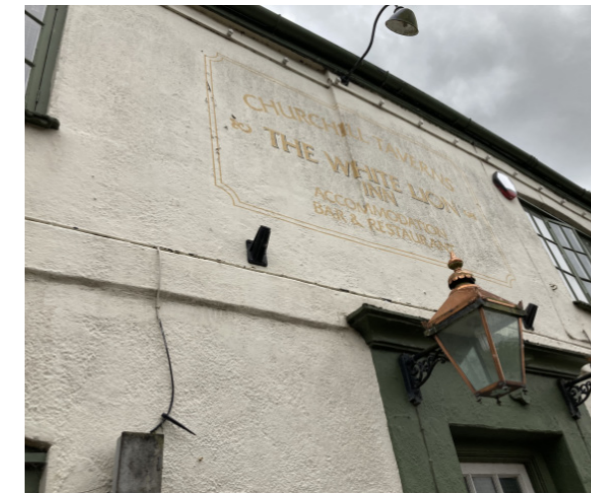
Vertical step in the frontage between the two 17th century phases of build.
