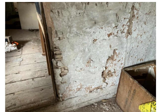
Above - original external timber frame at first floor level keyed to enable render to be applied. Below - split lathe and thick lime render to what was the external wall visible in the attic space.
