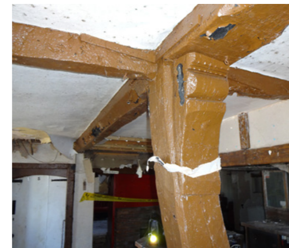
Vertical timber remains of the end wall at ground level with chamfers either side, that in the original phase is much deeper. Mortice holes from the original ground floor end wall visible.
