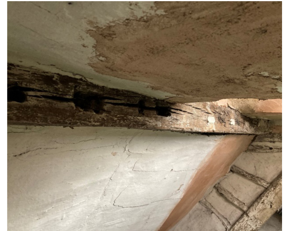
Above left - 17th century cellar door with blacksmith made hinges and shaped top. Above right – mortice holes in the underside of the purlin made from re-used timber close to the eastern dormer and round wood timber used to infill timber frame.
