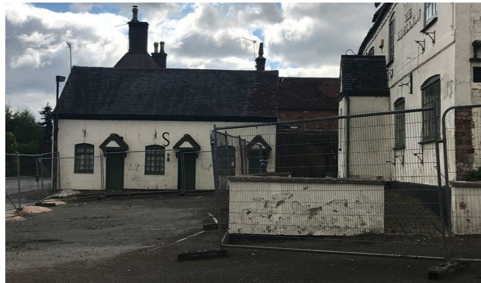
The Brewhouse East facade
