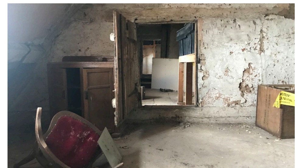
Existing second floor storage space
