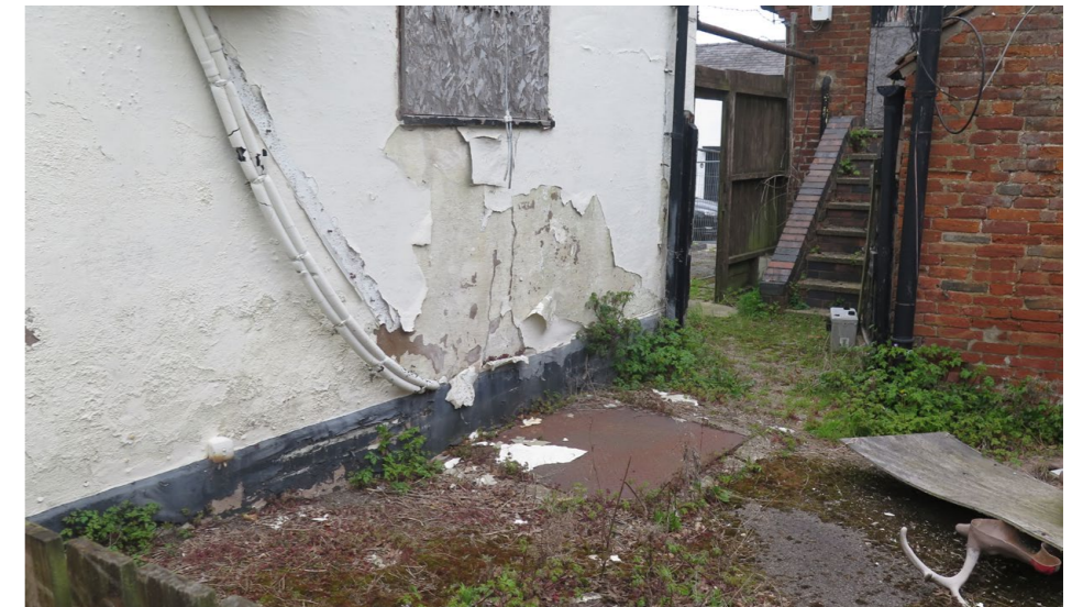
Existing trap door to the basement
