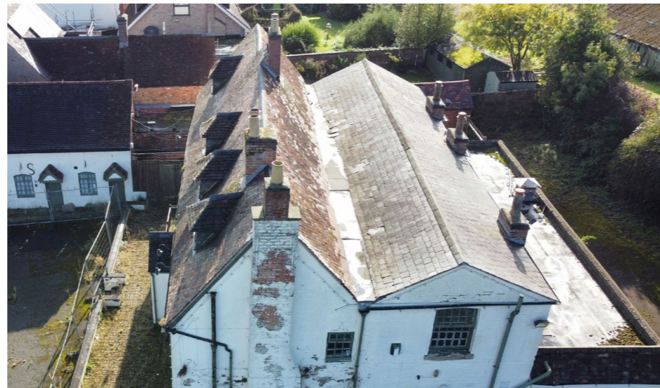
Existing clay- and slate-tiled roofs
