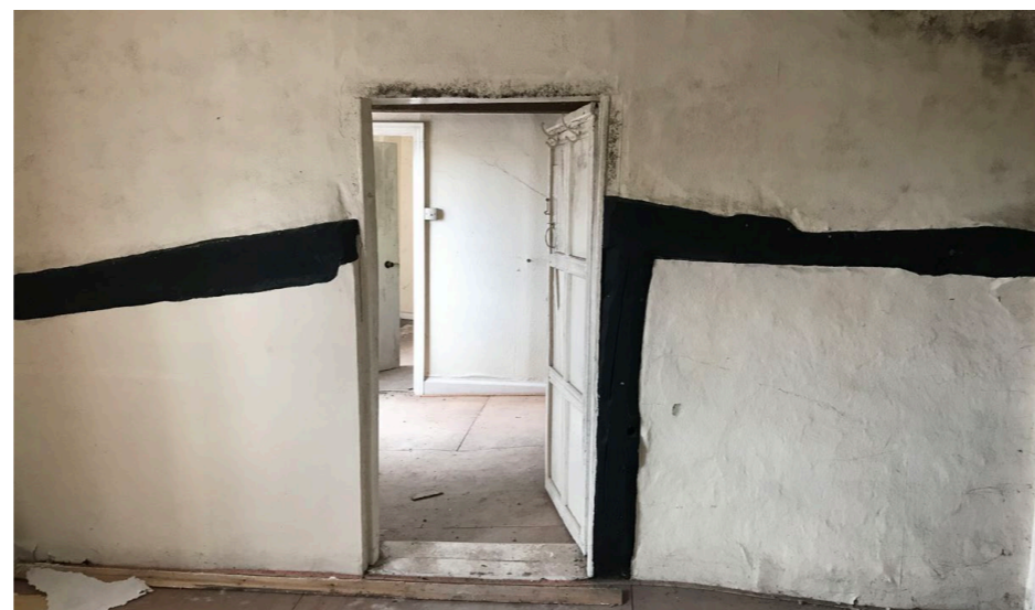
Existing first floor bedroom
