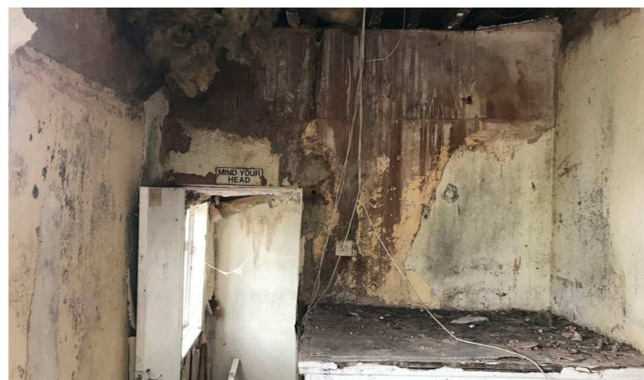
Existing first floor stair
