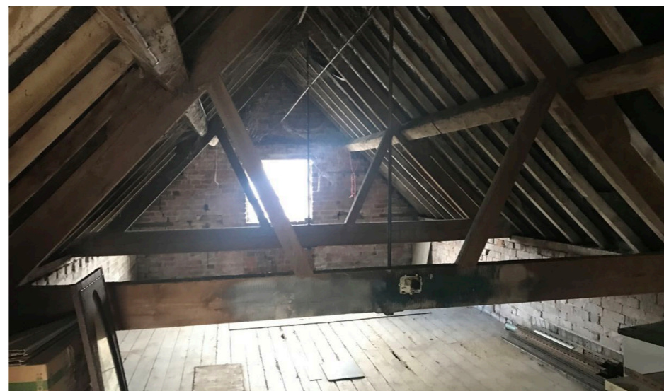
The Brewhouse existing timber roof structure
