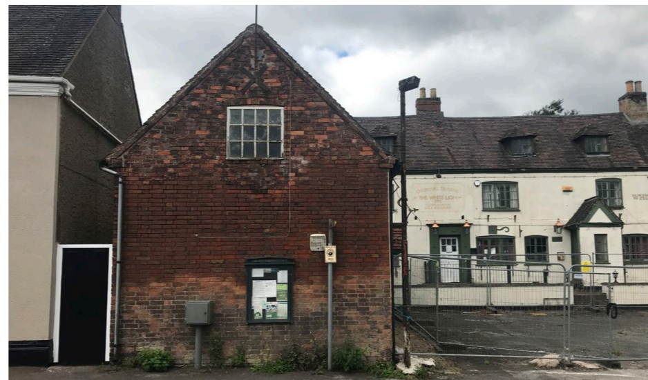
The Brewhouse North facade
