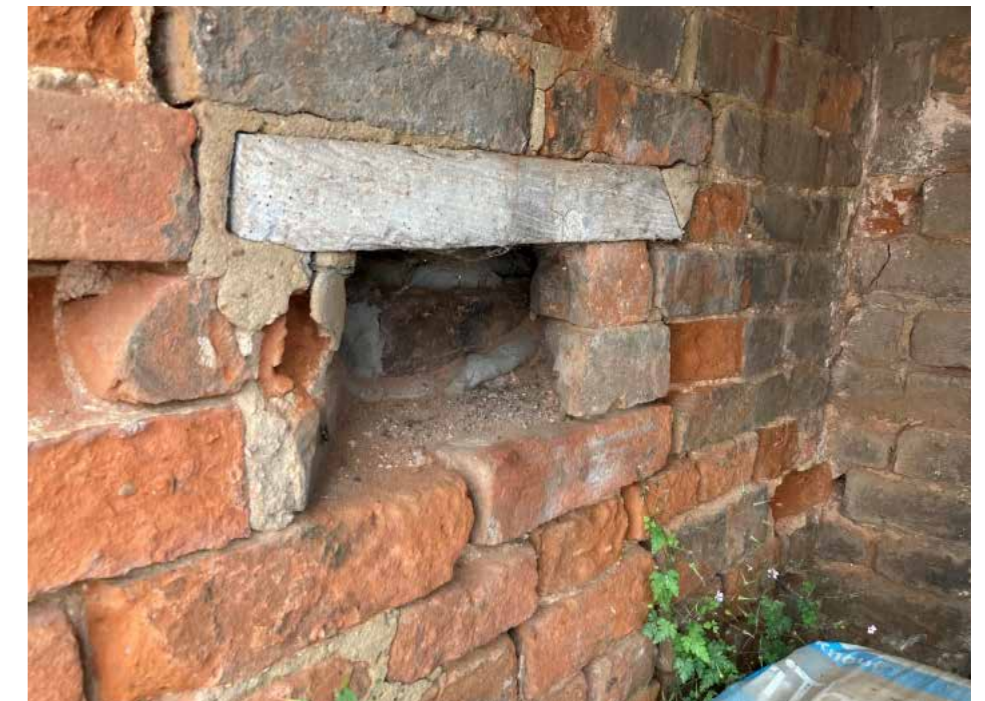
Above left – single storey brew house and two storeys outbuilding beyond – ventilation holes blocked by a single header can be seen either side of the iron cross at the top of the gable. Above right - stoke hole to fire the copper located within the brewhouse.
