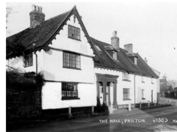
Exterior of the hall, Pailton. 1930s
