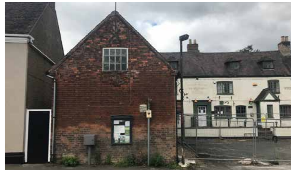
The Brewhouse North facade
