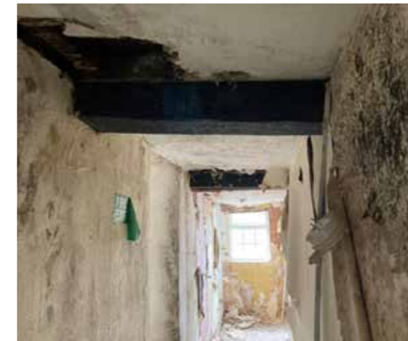
In the foreground, one of two new joists spanning the building front to back inserted to allow the rear access passageway to be cut through the timber frame, the second black painted "beam" is fake.
