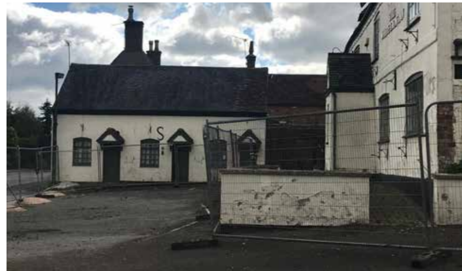
The Brewhouse East facade
