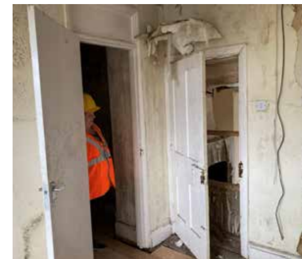
Mid-19th century door to allow access to the assembly room from the easterly bedroom.
