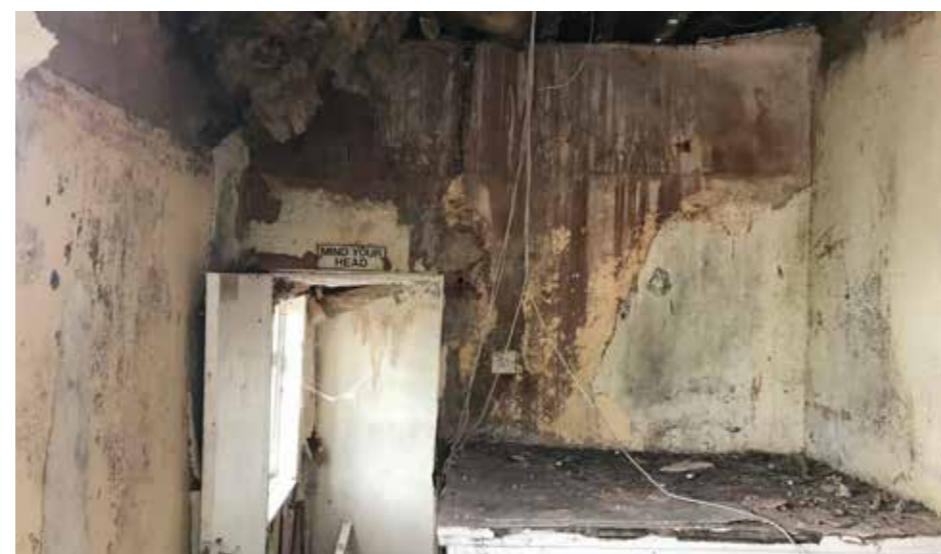
Existing first floor stair
