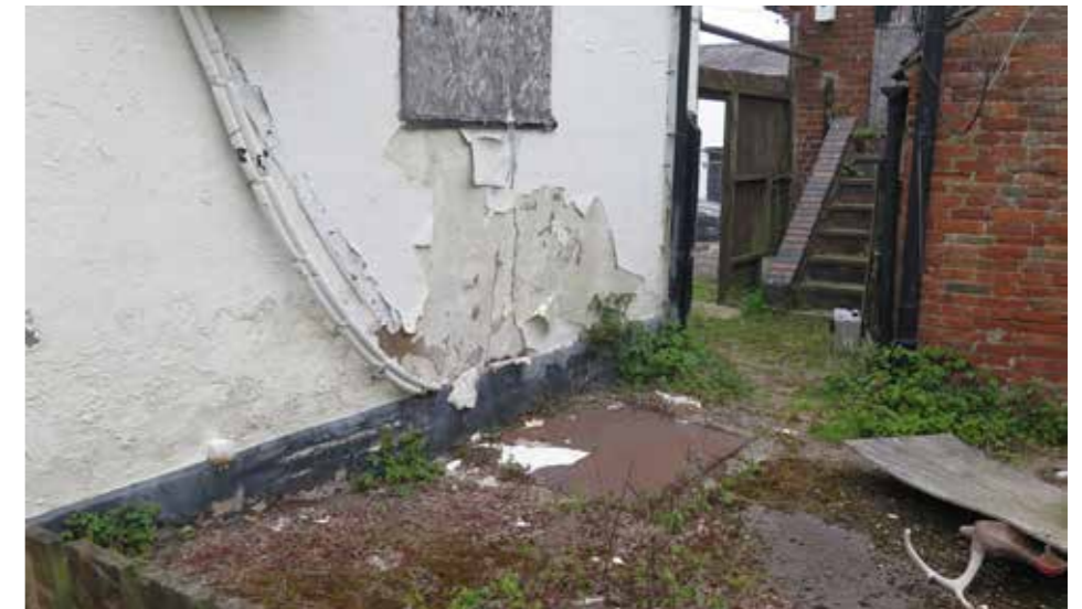
Existing trap door to the basement
