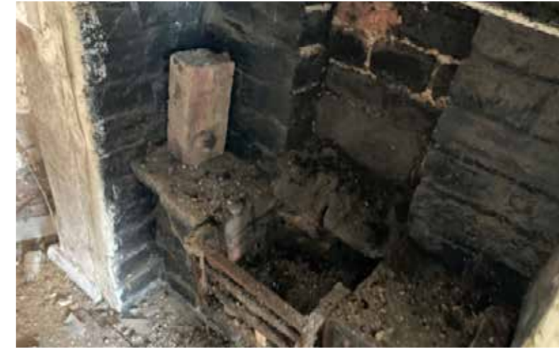
Left - possible frame to skylight in attic. Right - early 18th century fireplace in eastern most bedroom.
