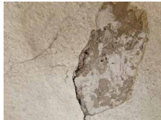
Above – apotropaic burn marks on inside end wall of the original timber framing. Below - specs of dark blue or black pigment of the lowest layer of limewash may be the remains of a decorative grisaille wall painting.
