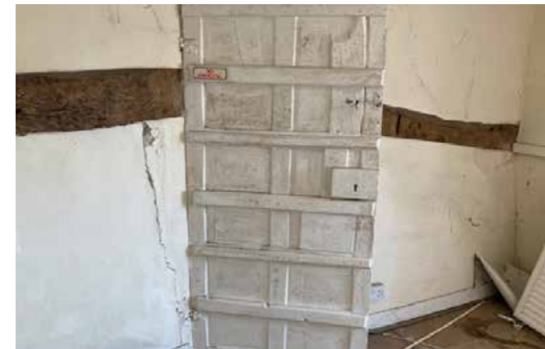
18th century six panelled door into new bedroom, the door is heavily re-enforced on the east side.
