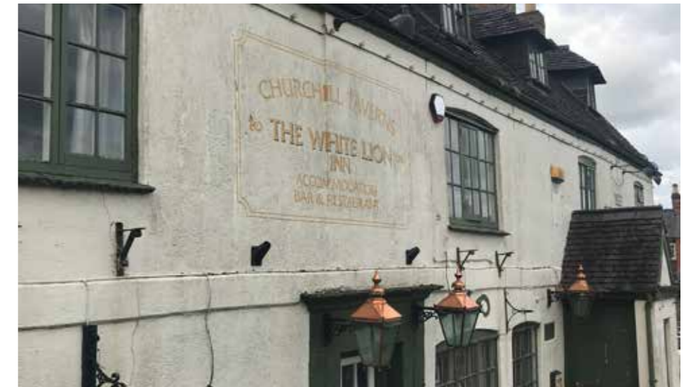
Existing front facade
