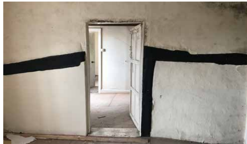
Existing first floor bedroom
