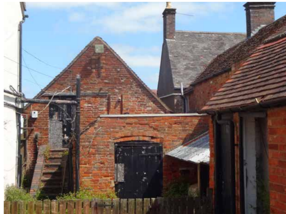
Above left – single storey brew house and two storeys outbuilding beyond – ventilation holes blocked by a single header can be seen either side of the iron cross at the top of the gable. Above right - stoke hole to fire the copper located within the brewhouse.
