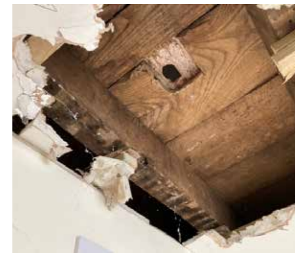
Limecrete over elm floorboards to create some sound proofing between the attic rooms and the bedrooms below.
