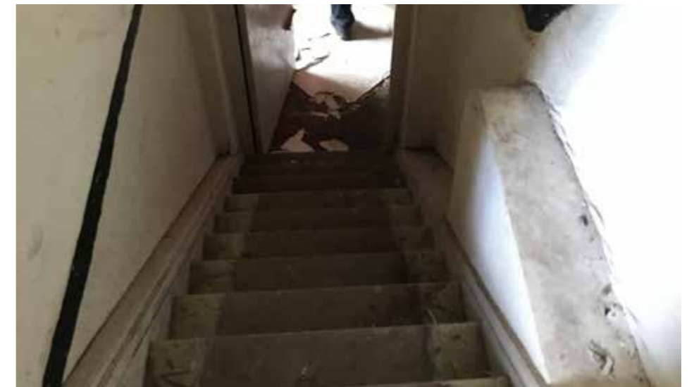
Existing historic stair
