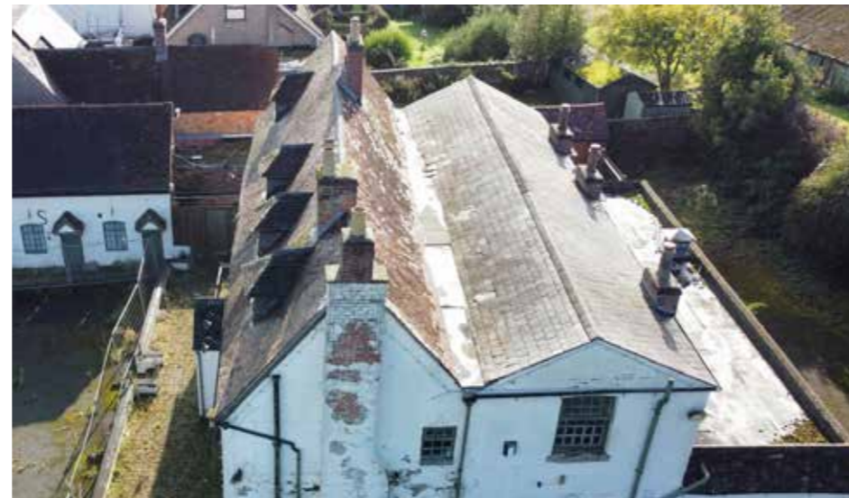
Existing clay- and slate-tiled roofs
