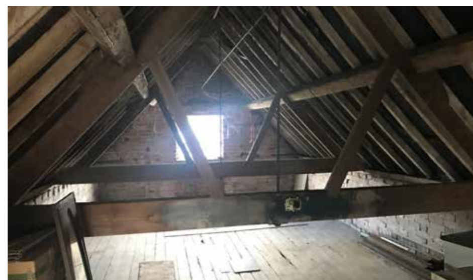
The Brewhouse existing timber roof structure
