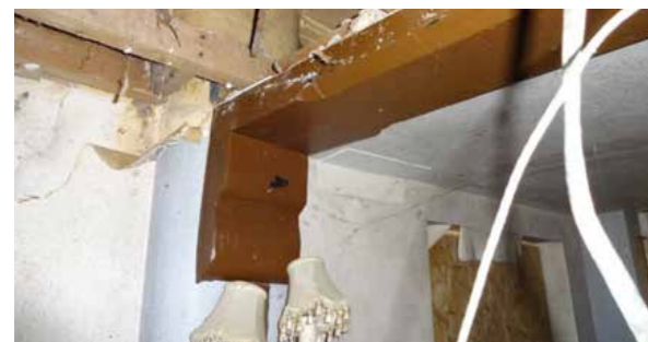
Post 1986 fake beam with chamfer, stop and a carpenter's mark with a false ceiling added below to what had been the upstairs assembly room, later converted into the landlord's flat
