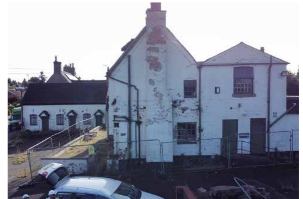
West facade and existing forecourt
