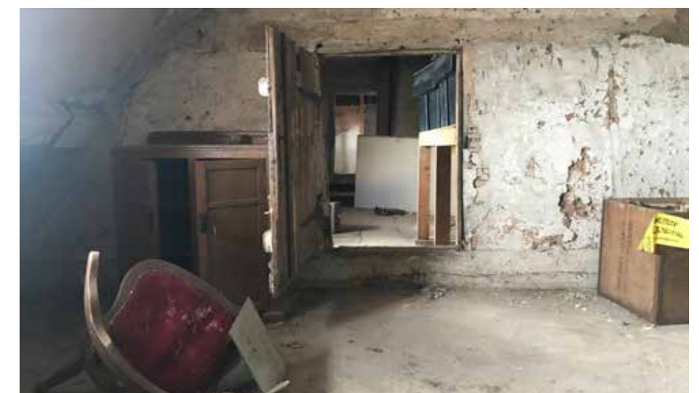
Existing second floor storage space
